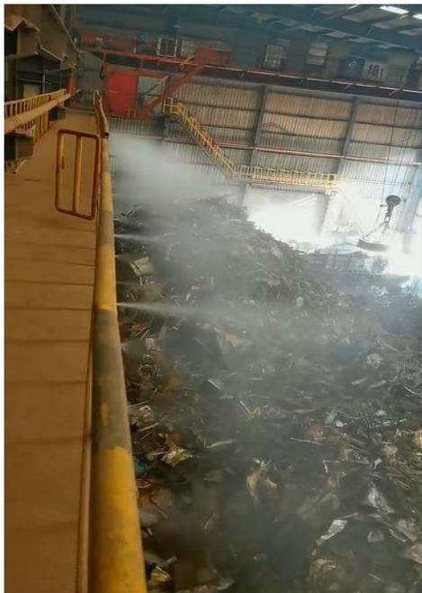
炼钢车间原料棚装卸上料区喷雾抑尘 1
